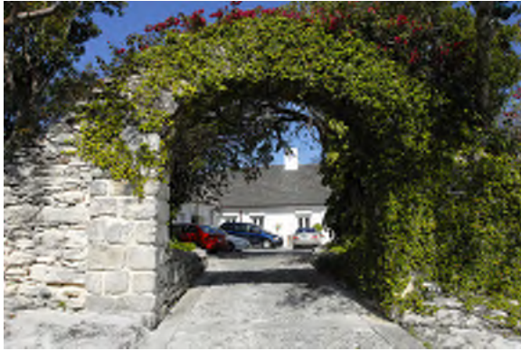
THE HEAVIER THE MATERIAL, SUCH AS THIS STONE WALL AND ARCH, THE MORE SENSE IT MAKES TO ACQUIRE IT LOCALLY
