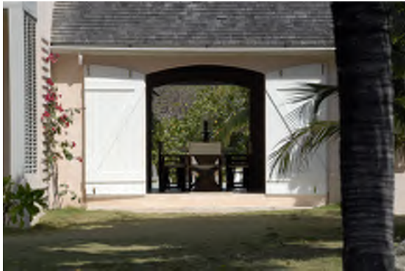
BUILDINGS WITH THIN WINGS ALLOW MORE ROOMS TO OPEN DIRECTLY TO THE OUTDOORS
