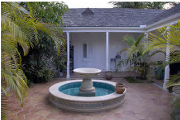
COURTYARDS OCCUR ONLY WHEN WINGS OF THE BUILDING ARE MADE THIN ENOUGH AND LONG ENOUGH TO CREATE THE COURTYARD SPACE
