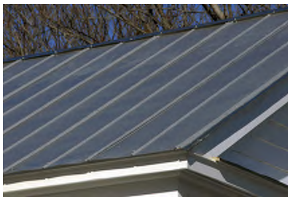
5V CRIMP METAL ROOFS REFLECT MOST OF THE SUN'S HEAT BEFORE IT EVER ENTERS THE BUILDING.
